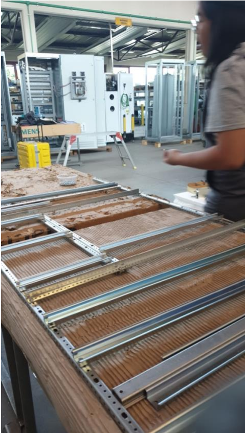
Picture 5: On the Job
